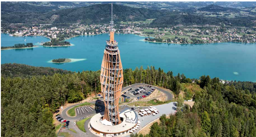
Photos © Rubner Holzbau
