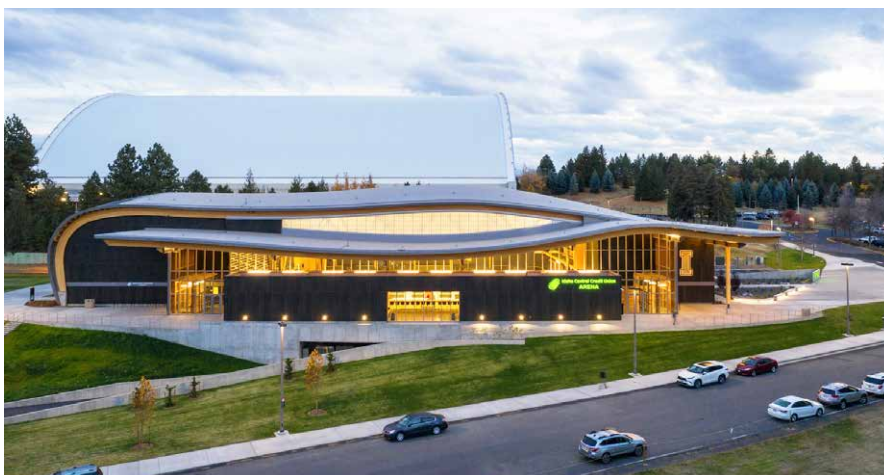
Photos © Structure Craft
